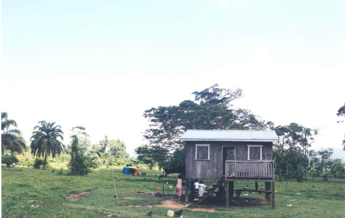
Figure 16. Traditional house with tin roof
